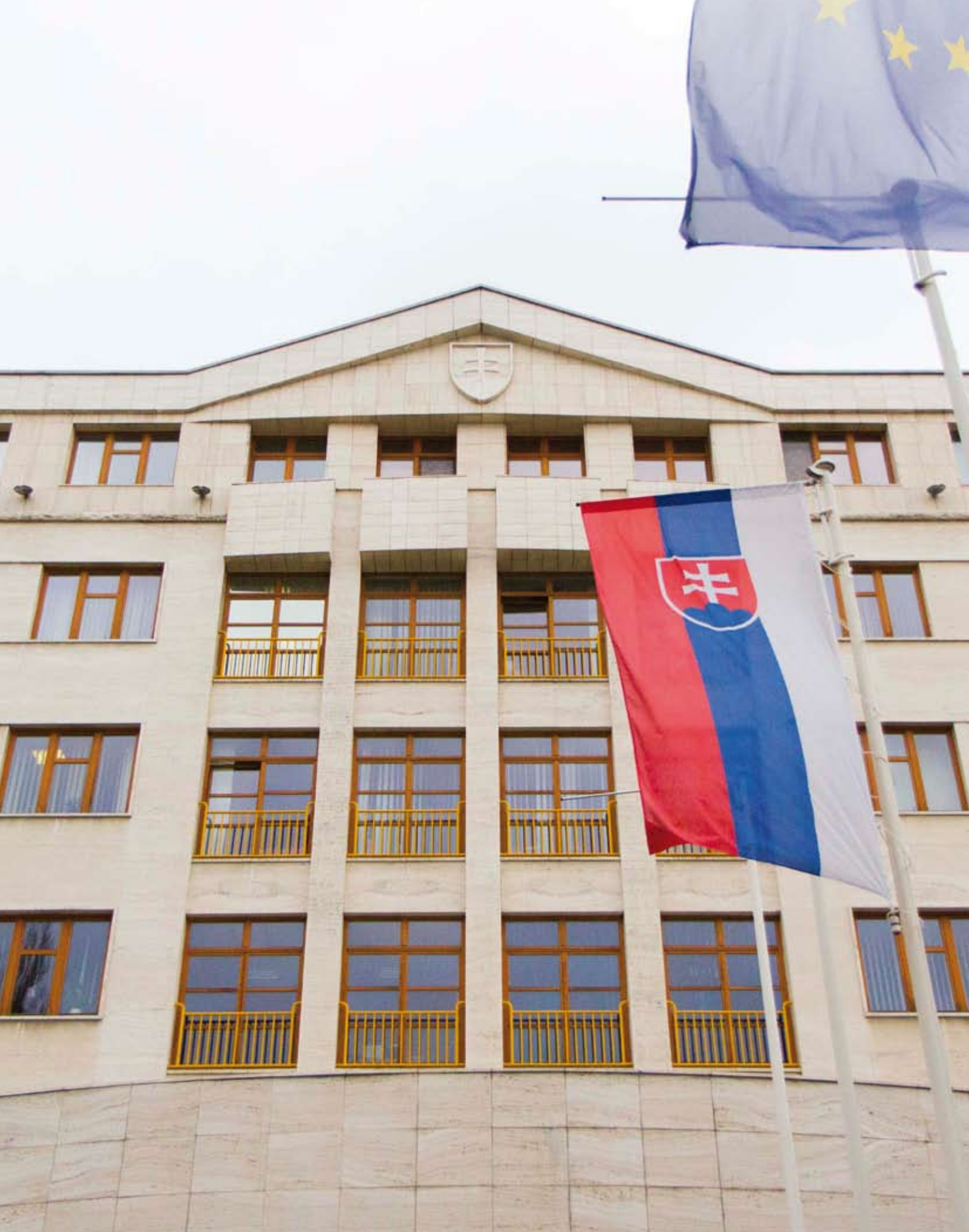
Building of the Ministry of Foreign and European Affairs of the Slovak Republic (Photo: MFEA SR)
