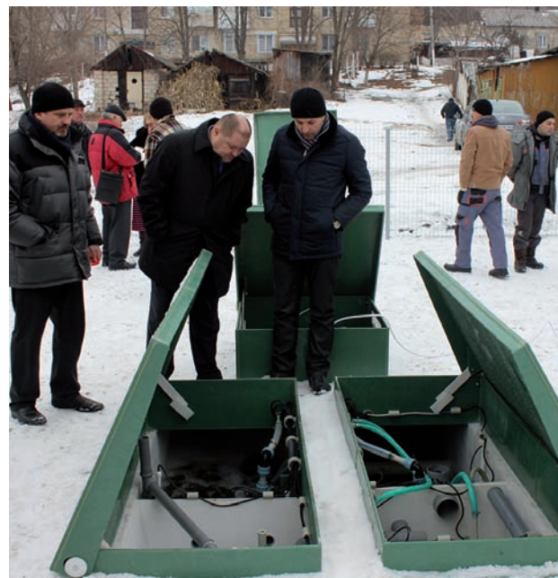
▲ Building a sustainable waste water treatment system in the Moldovan village of Bucovăț (Photo: SlovakAid/Peter Tomášek)
