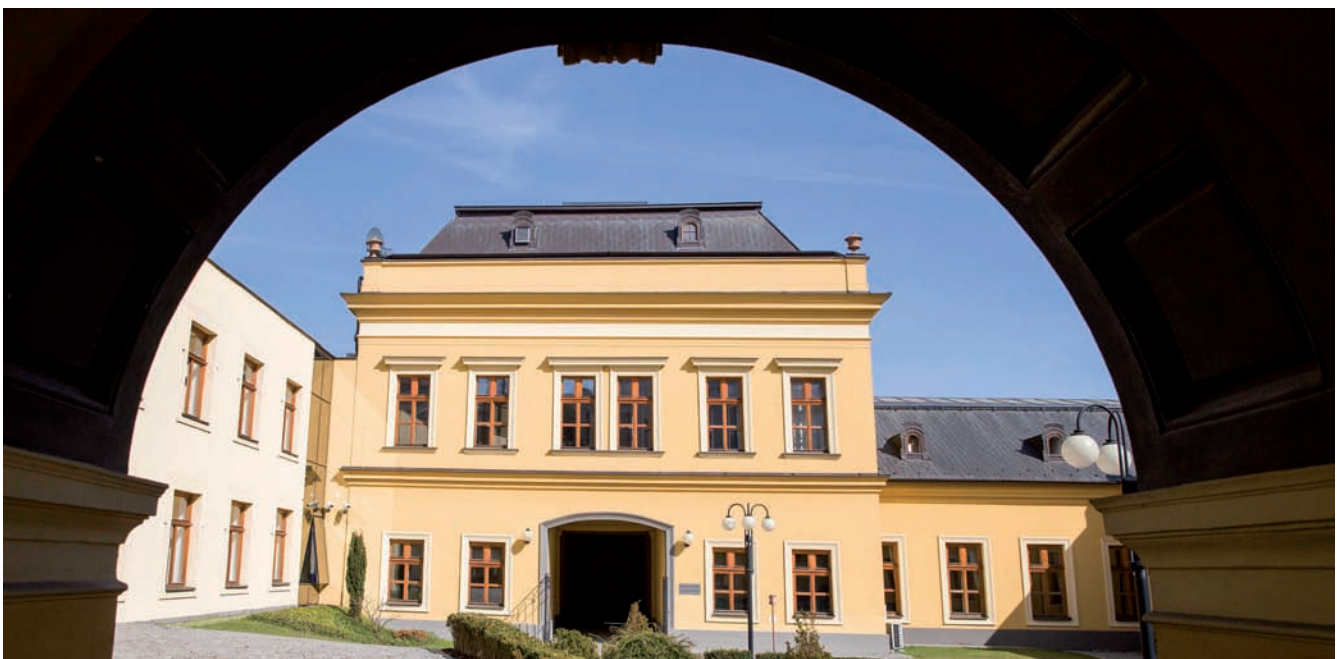
▲ Palugay Palace – a building of the Ministry (Photo: MFEA)
